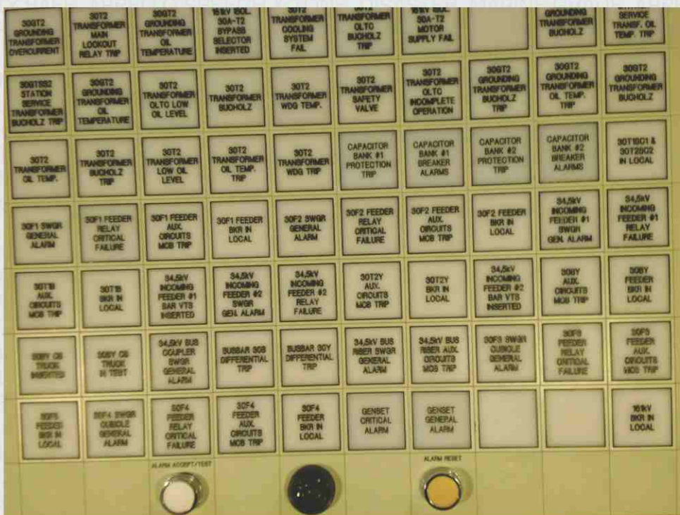
Ghana Mimic showing Multi 16 units with 48x48mm Mosaic display
